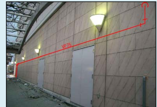
A pipe will be laid on the wall.
