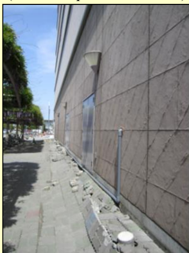
(Before improvement work)
