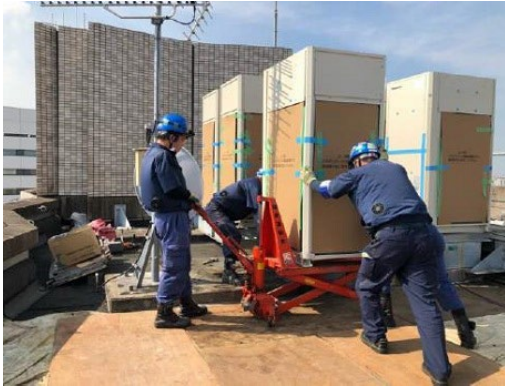
upgrading of air-conditioning systems (Courtyard by Marriott Shin-Osaka Station)
