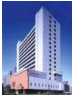
Nissan Motors New Headquarters Bldg.
